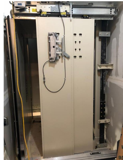
DME has installed the elevator cab!
